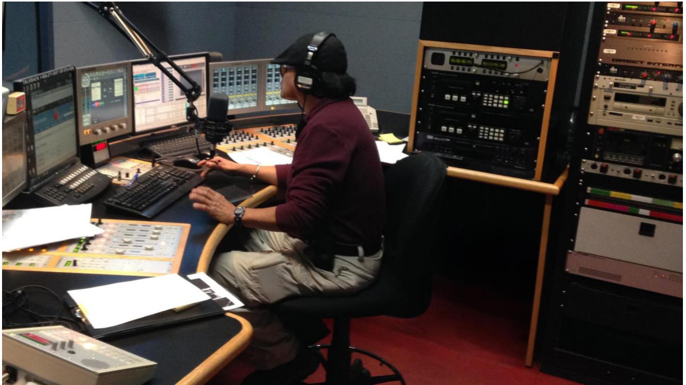
Our broadcast control room in Yellowknife.
